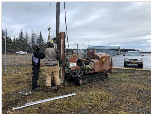
Exhibit 4-1: Drilling near the Alaska Airlines terminal
