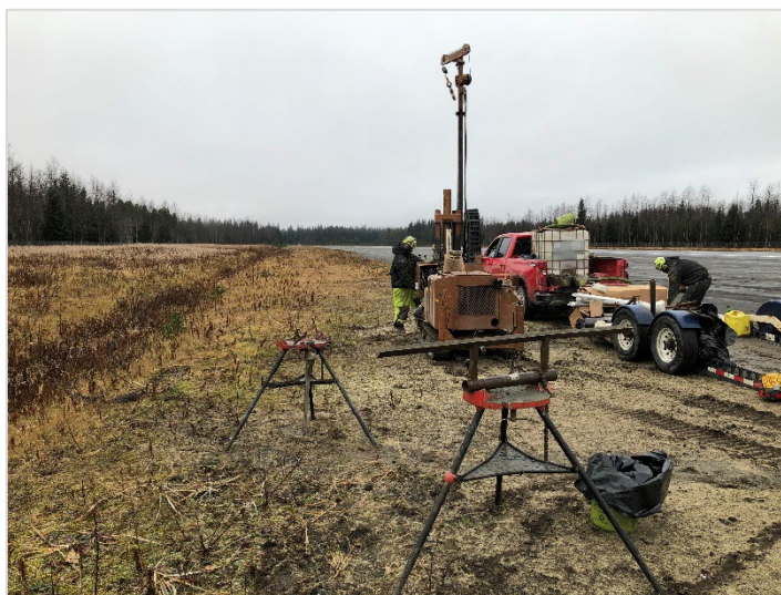
Exhibit 2-1: Drilling at Runway near the ARFF building
