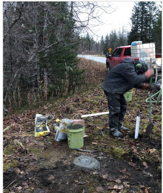
Exhibit 2-2: Well installation at MW-22
